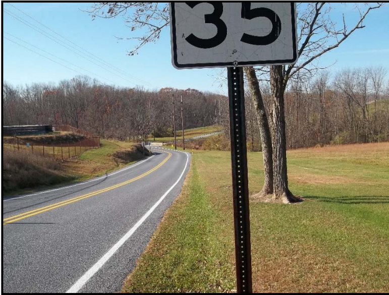
Photo 16 (11-10-2014) View of Coulter Road at the southern end of the project study area. View is west.
